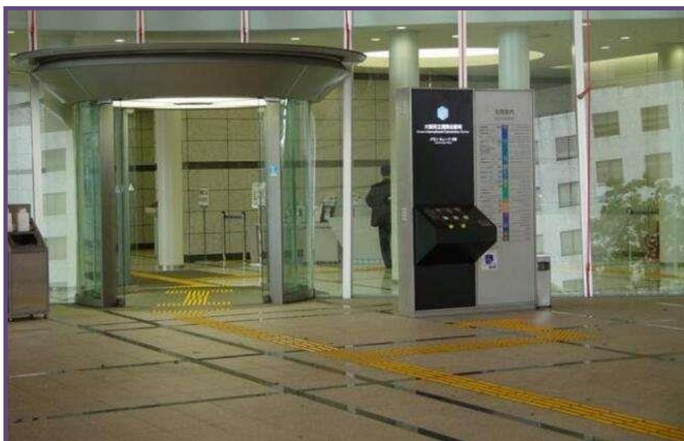
Photo 4-1. Accessible Main Entrance with Tactile Pavers
