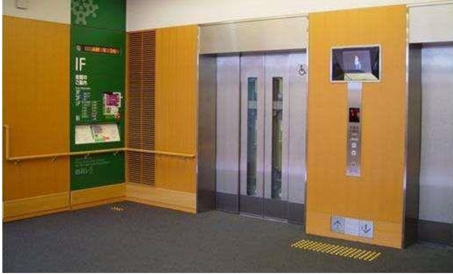
Photo 10-1. Lift signage and colour contrasted amenities
