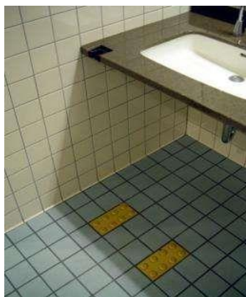
Photo 15-1. Floor Markings with Warning Pavers for Persons with Visual Impairments
