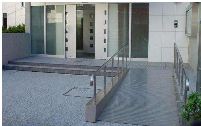
Photo 7.1 Combination of ramp and steps
