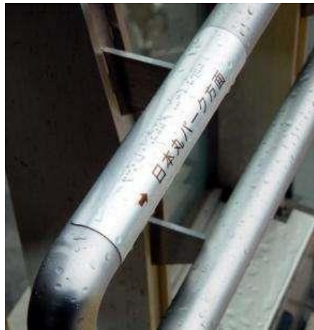
Photo 9-1. Handrail with Braille Information
